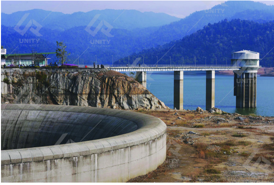
BUKIT SAH WATER TREATMENT PLANT , KEMAMAN
