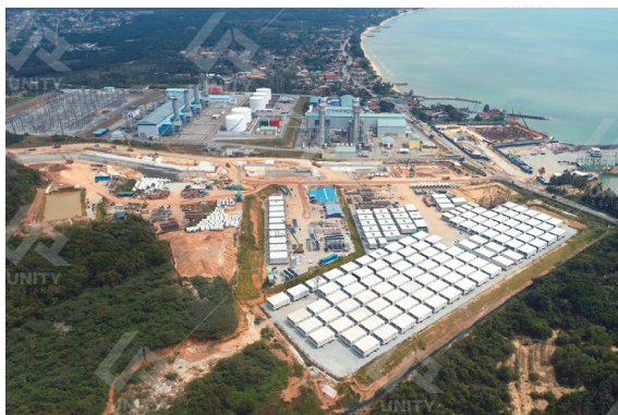
MELAKA CCGT POWER PLANT
